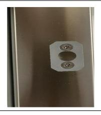
10. Move the lock fitting from the former top edge to the intended top edge of the door.
