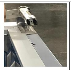
11. Place the door closer at the bottom left at an opening angle of 180°, and put the bottom left corner of the door over the door closer with the recess provided.
