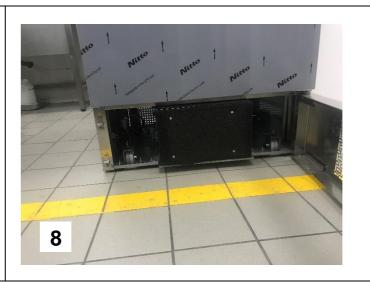
7-8) The lower front plate which is designed with magnet of the cabinet can be easily open/close and reachable.
