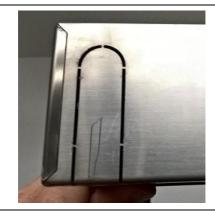
14. Break out the left recess at the bottom of the canopy flap.
