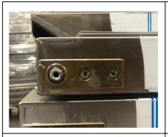
7. Remove the door closer without turning the door closer square.
